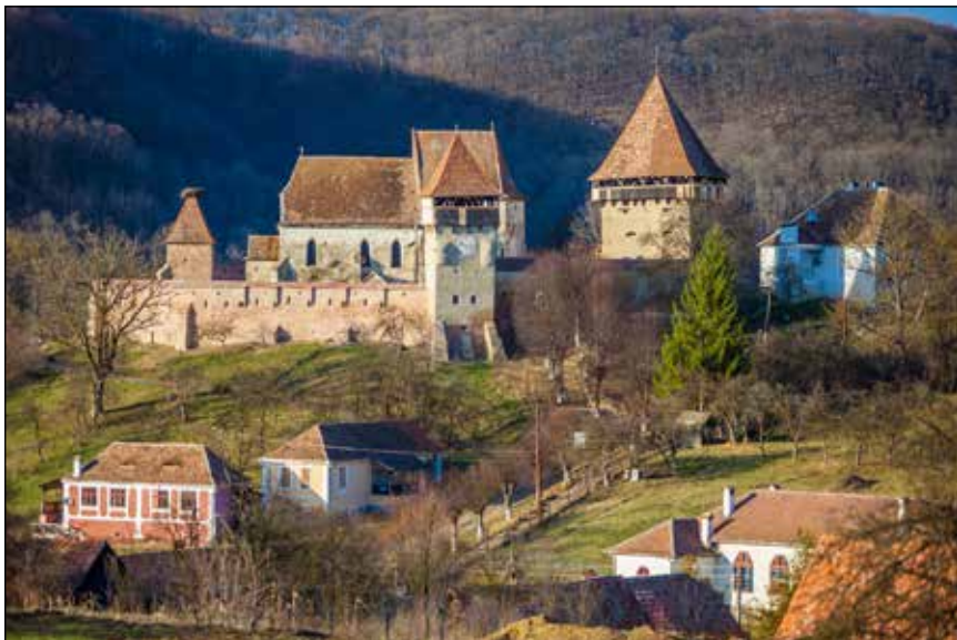
■ Foto 2. Alma Vii, cetate fortificată după restaurare © MET ■ Photo 2. Alma Vii, fortification after conservation © MET
